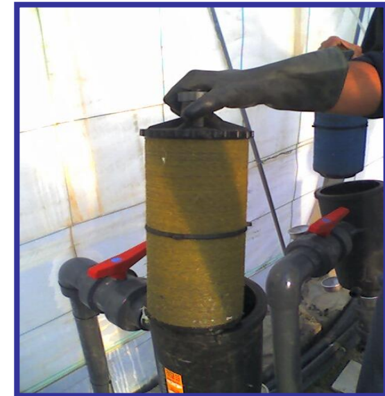
Frequent maintenance of the filters
